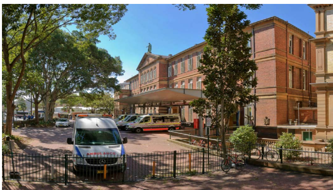
Figure 2. The Albert Pavilion Royal Prince Alfred Hospital 2016.
